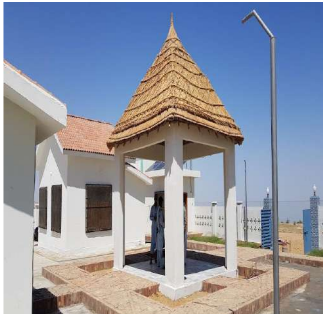
Manchar Lake Resort 2 Rooms
